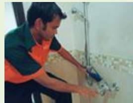
Plumbing and Pipe Repairs
