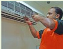
Air Condition Maintenance
