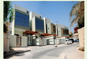
33 Units 2-Storey Villa in Mahooz
